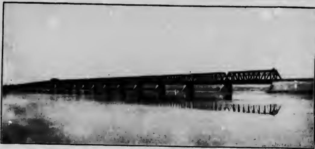
Grand Trunk Railway system—Victoria Bridge, Montreal.
