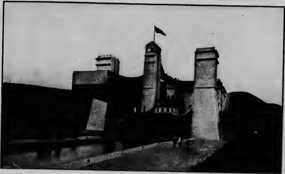
Hydraulic Lift Lock—Peterboro', Ont. Vertical . . . 66 feet. The largest in the world.
