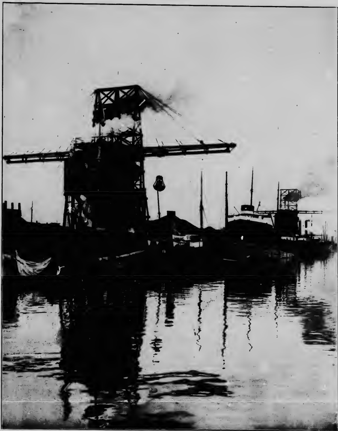
Nova Scotia Steel and Coal Co.—Discharging and bunkering plant at Quebec.
