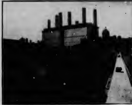
Montreal Harbour Commission—Elevator No. 2 in course of construction.
