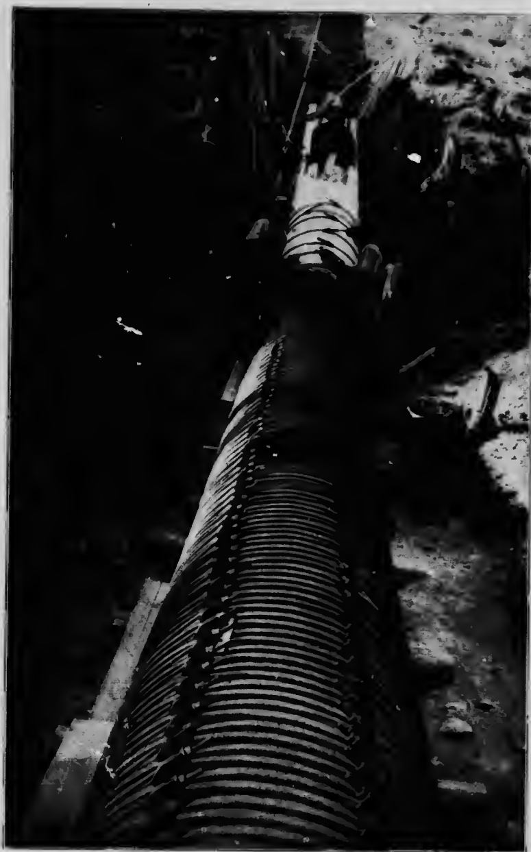
White Valley Irrigation and Power Co. Ltd., Vernon, B.C.—36-inch continuous wood-stave pipe, B. X. Creek.
