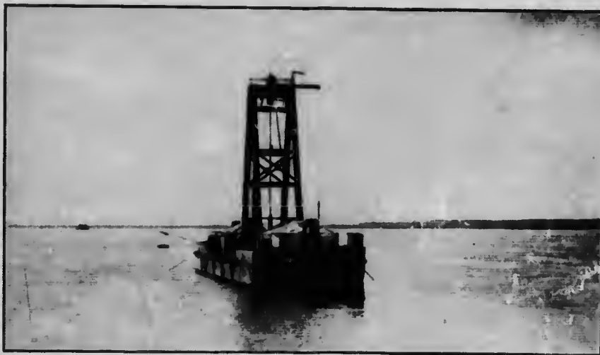
Twenty ton rock cutter working at Cap-à-la-Roche St. Lawrence river.
