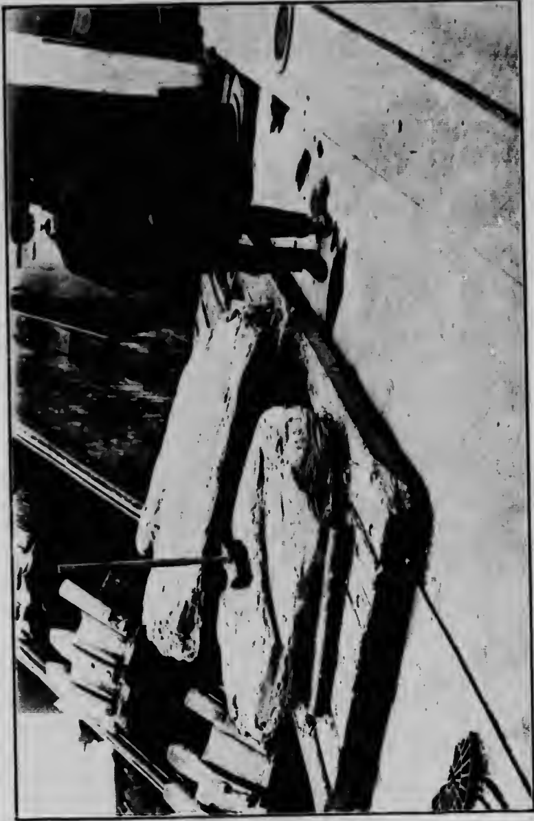
Shale rock dredged by Dredge No. 3 at Cap St. Charles, without the aid of explosives.
