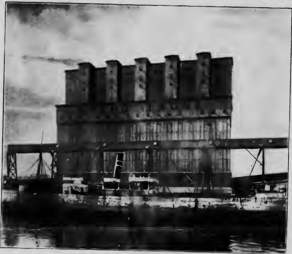
The Grand Trunk Elevator, Montreal.
