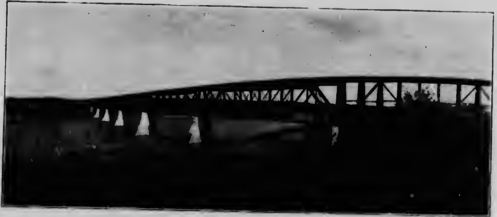
Canadian Northern Ry.—Fenton Bridge, across Saskatchewan river.
