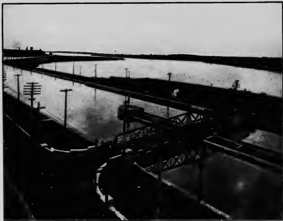
Cornwall Canal—Swing-bridge at Cornwall.
