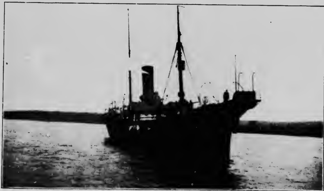
Canadian Government steamer "Lady Laurier," with cable laying apparatus.
