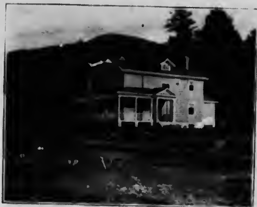
Lighthouse and buoy depot, Prince Rupert—Residence of the official in charge.
