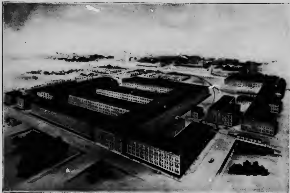
Canadian Westinghouse Co. Ltd.—Works at Hamilton, Ont.
