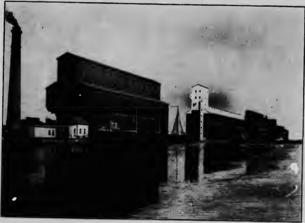
Canadian Pacific Railway Company—Grain elevator at Fort William, Ont.
