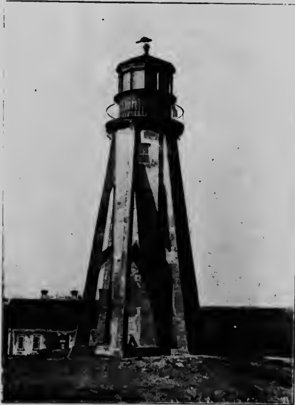
Reinforced concrete tower with flying buttresses, well-known type of Canadian lighthouses.
