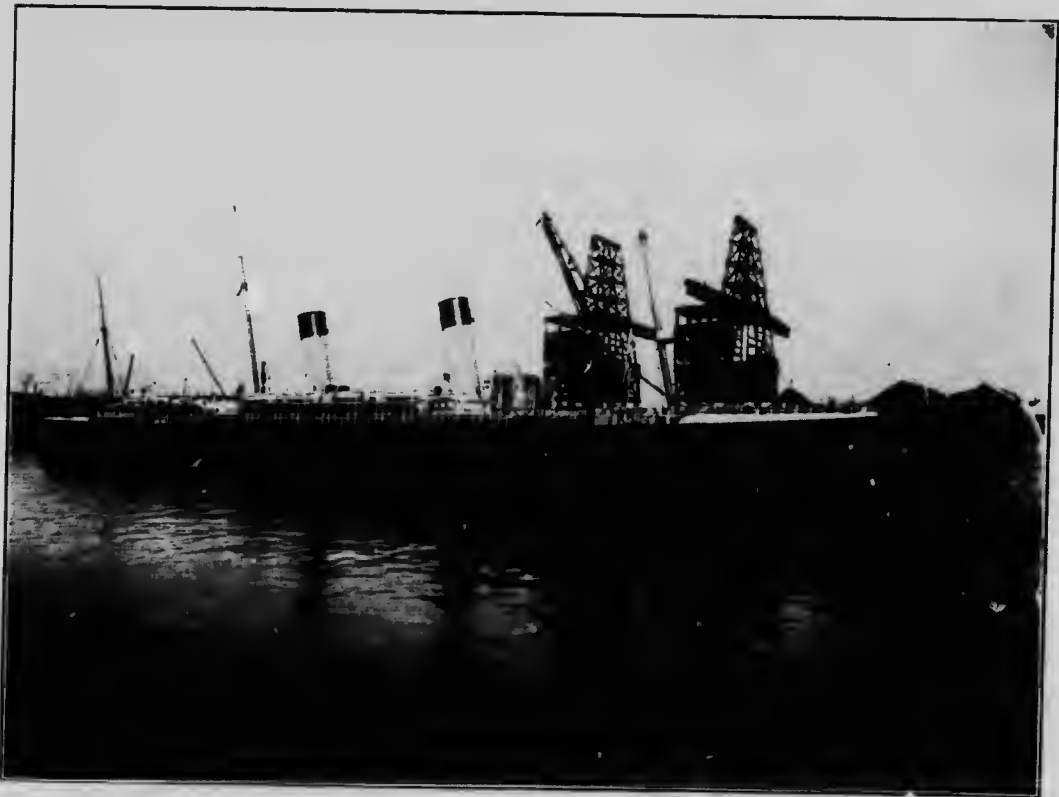
Montreal—S. S. "Teutonic" bunkering at Nova Scotia Steel and Coal Co.'s coal towers
