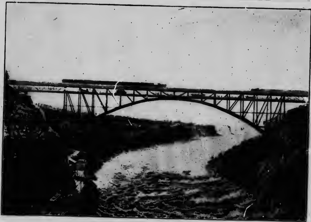
Grand Trunk Ry. system—Steel arch bridge across Niagara gorge.
