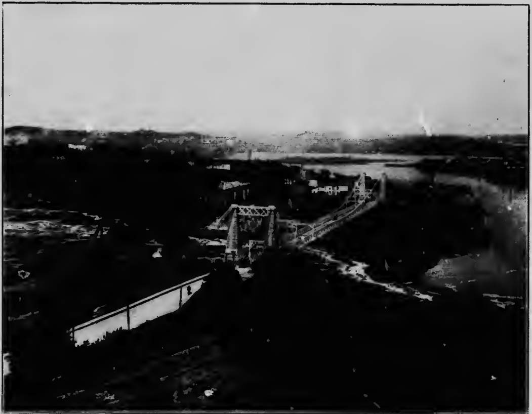
Intercolonial Railway—Entrance to St. John, N.B.
