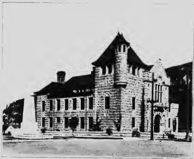
Kaslo marble. Court house, Nelson, B.C. (The monument to the left is of Nelson granite from Three-mile point, Kootenay lake.)
