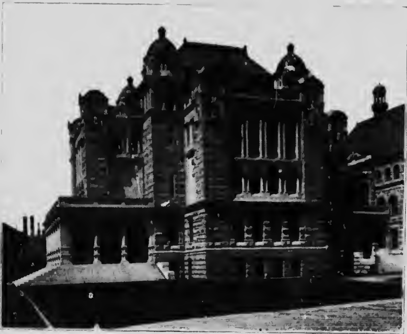
Haddington Island andesite. New library, buildings of the Legislative Assembly of British Columbia, Victoria, B.C.
