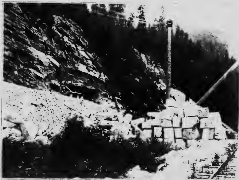
Marble blocks and portal of quarry of the Canadian Marble and Granite Works, Marblehead, B.C.
