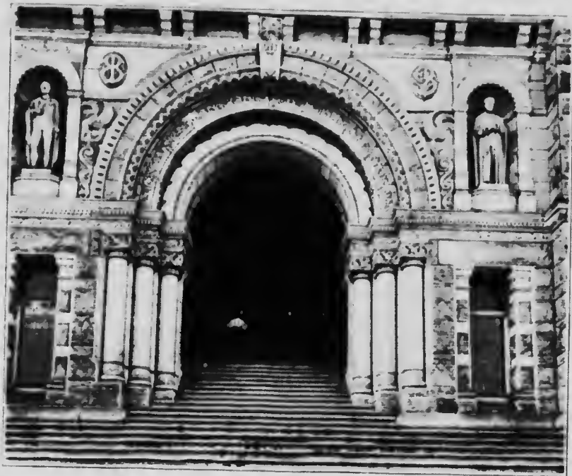
Haddington Island andesite. Main entrance, buildings of the Legislative Assembly of British Columbia, Victoria, B.C.
