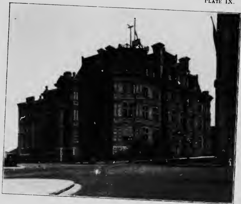
Gabriola Island sandstone. Post-office, Victoria, B.C.
