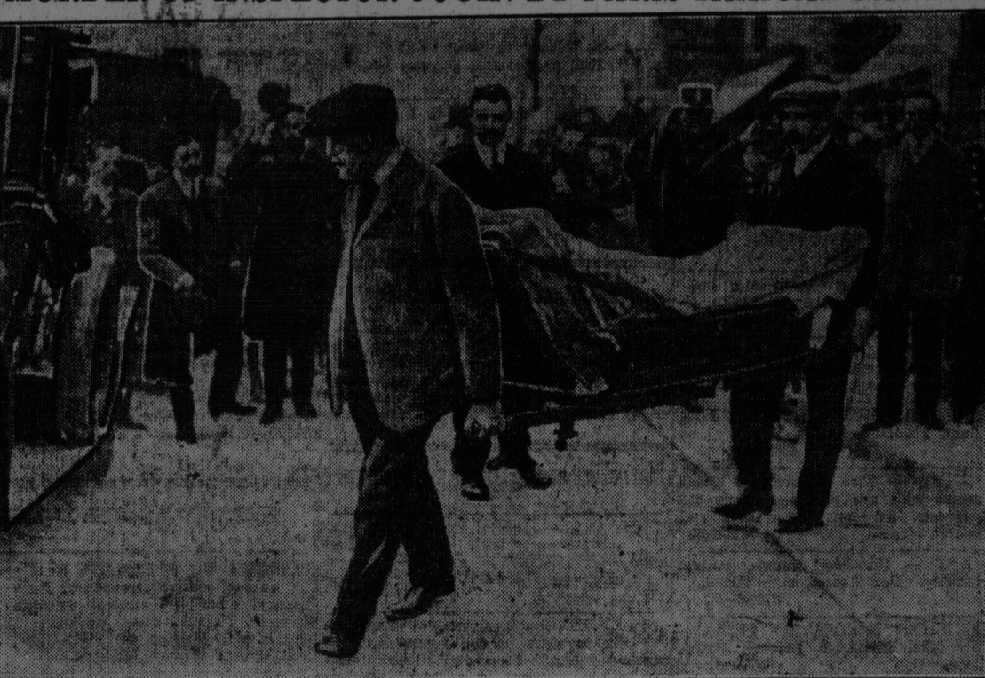
This shows the body of the assassinated Jouin being carried from the house where he was shot and killed by Bennet, the leader of the bandits, who lured the detective into a house on the pretense of giving information. While ascending the stair Jouin was shot by the bandit inside. The murderer was subsequently killed in a running fight with the police and soldiers.
