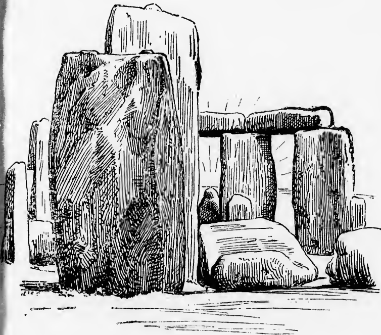
FIG. 37.—Trilithons and other Stones at Stonehenge. Notice the projections on the top of the large upright stones, which fit into corresponding depressions on the under surfaces of the imposts. (From Barclay's "Stonehenge.")
