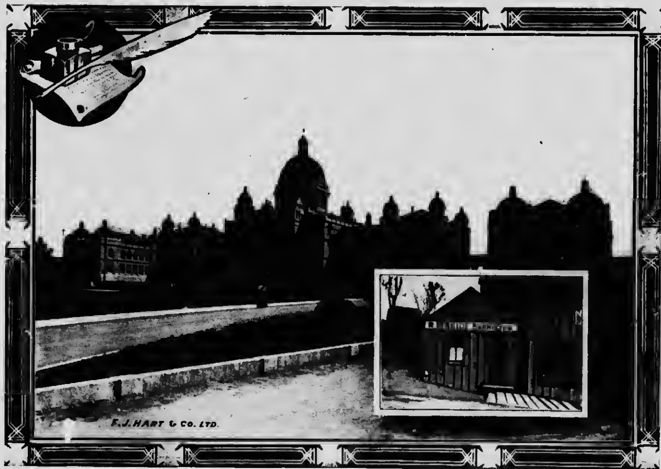
(INSERT) LAW OFFICE OF RICHARD McBRIDE, NEW WESTMINSTER, B. C., IMMEDIATELY AFTER GREAT FIRE OF 1898. BRITISH COLUMBIA PARLIAMENT BUILDINGS, VICTORIA, B. C., 1911. HON. RICHARD McBRIDE, PREMIER.
