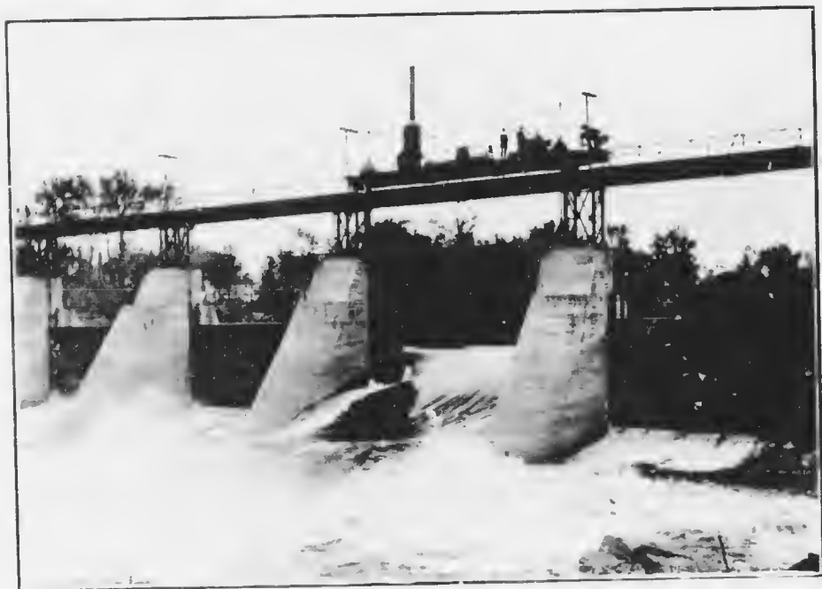
The Saint-Maurice dam at Shawinigan, seen closer.
