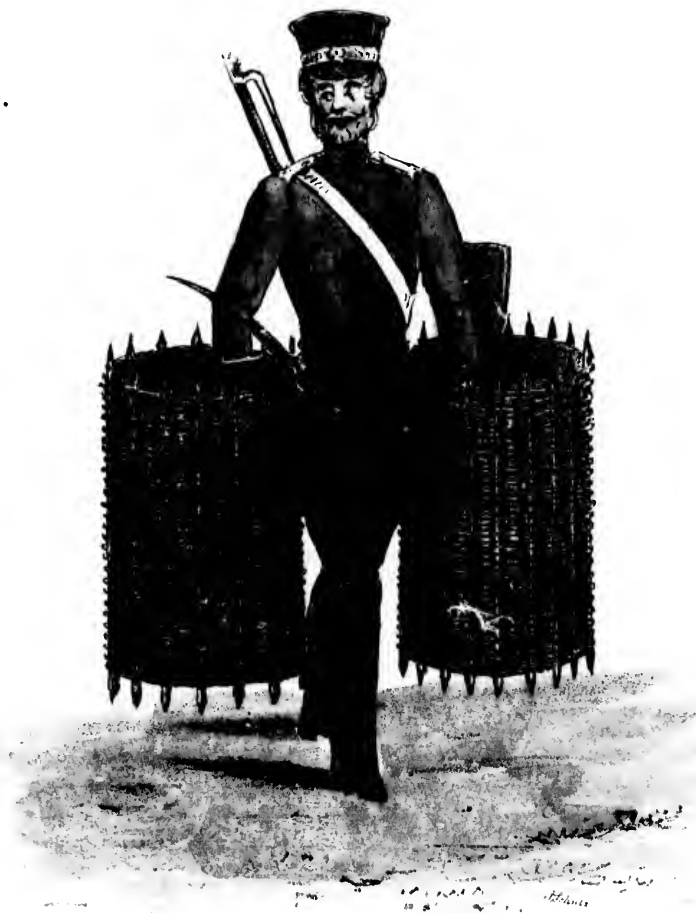
Sketch showing the method of carrying the Gabions in advancing to make a Flying Sap.
