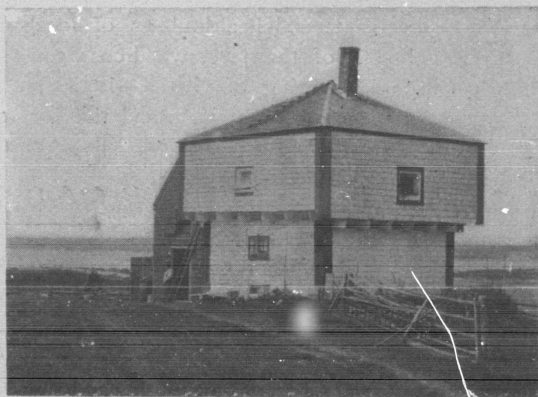
THE BLOCK-HOUSE, BUILT 1812, ST. ANDREWS
