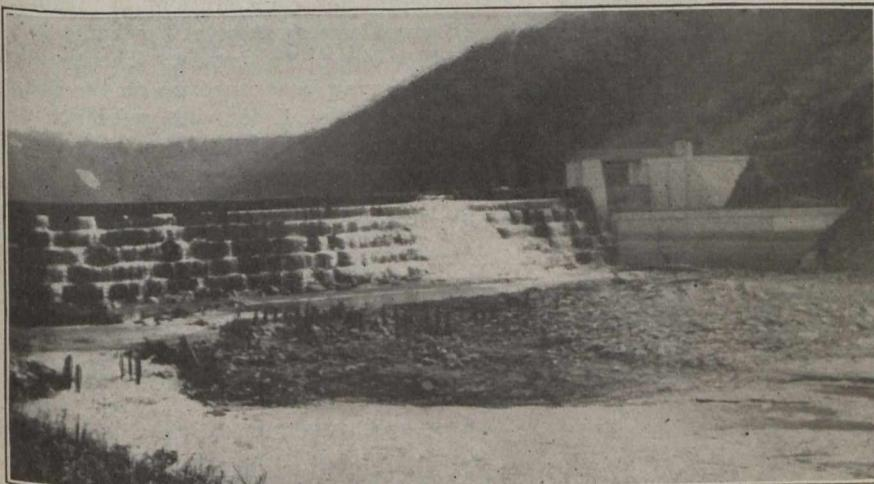
Loch Raven Tilting Dam, Showing One Section Held in Open Position by an Obstruction at the Toe. Water Surface Elevation, 191.5 Ft.
