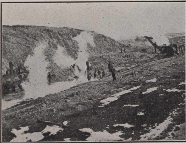
Fig. 3.—Inefficient Drilling Due to Clouds of Steam.
