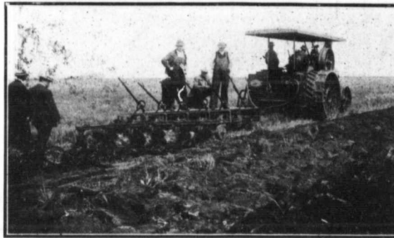
Pulling 6-14 in. Breaker Bottom Plows—Delivering 30.76 Draw-Bar Horse Power Draw Bar Pull Averaged 4,950 pounds—825 pounds per plow.
