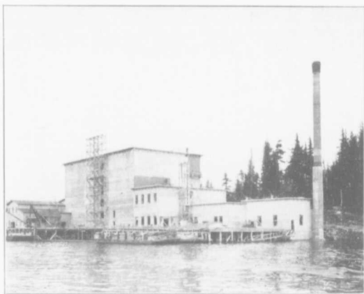
Rupert's Cold Storage Plant—Largest Single Unit Plant on Continent.
