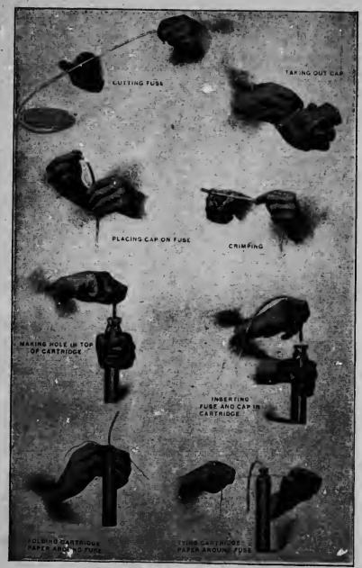
Priming a dynamite cartridge in the end.
