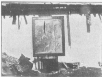
COURT ROOM AFTER THE FIRE.
