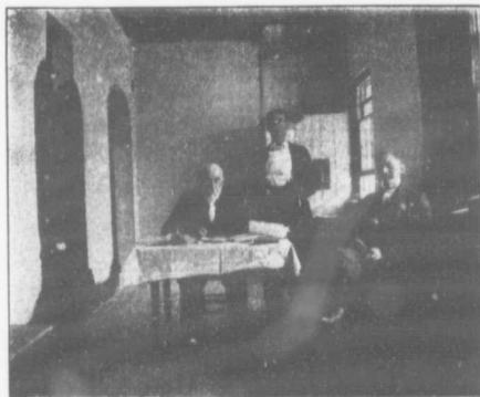
F. HUNT, J. P., HOLDING COURT IN A GAOL WARD, AFTER THE FIRE.
