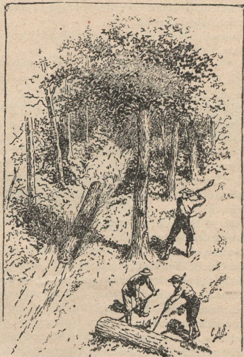
CUTTING TIMBER FOR RAFTING.
