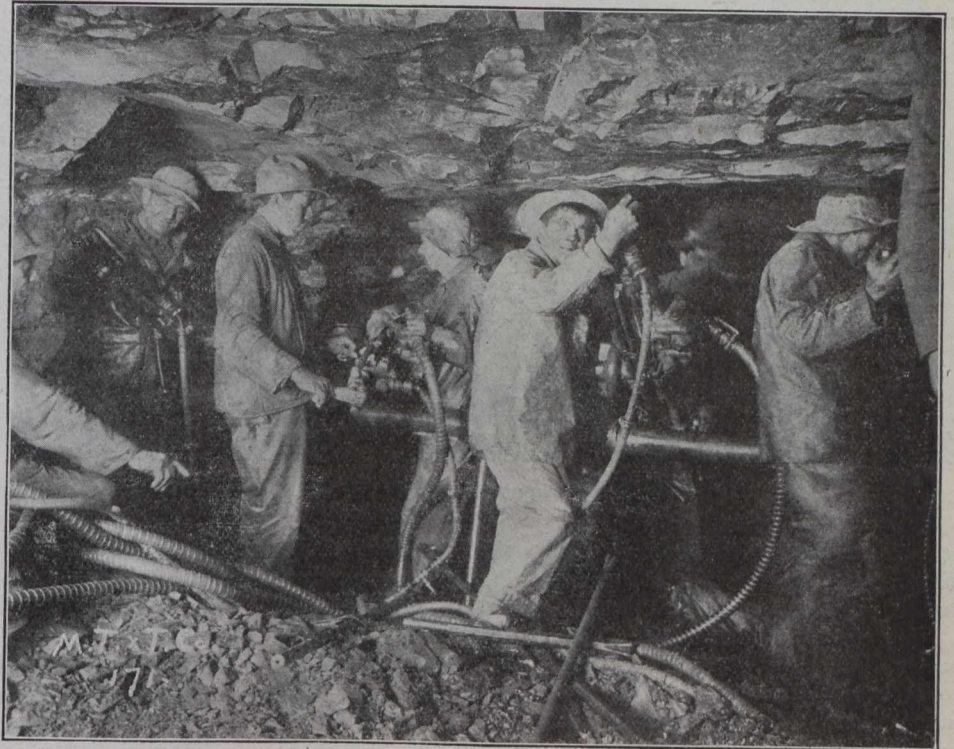
Fig. 1.—Face of Leading, Showing Rock Drills Mounted on Horizontal Bar.
