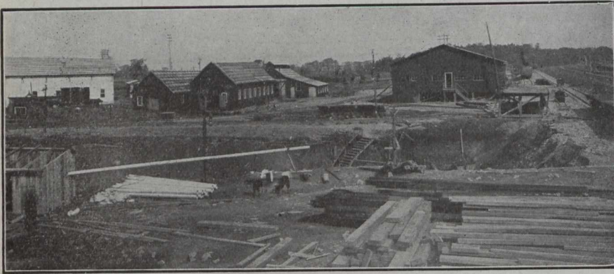
Fig. 3.—Western Approach to the Tunnel.
