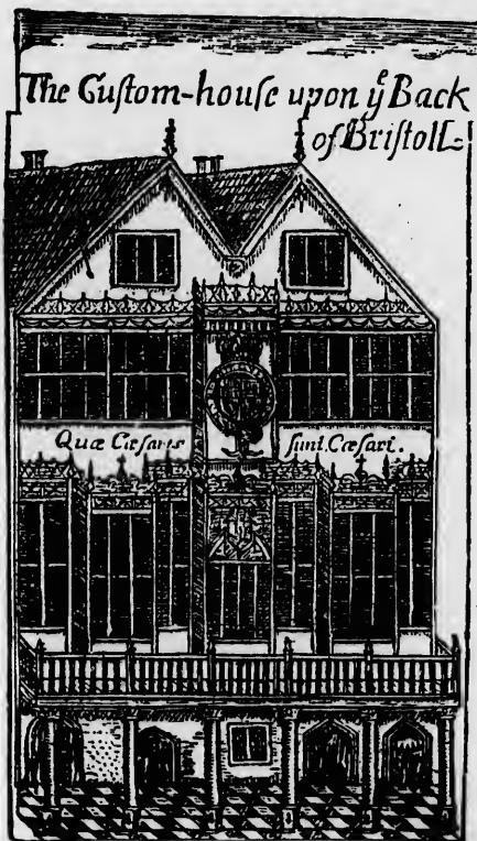
CUSTOM HOUSE, BRISTOL.
