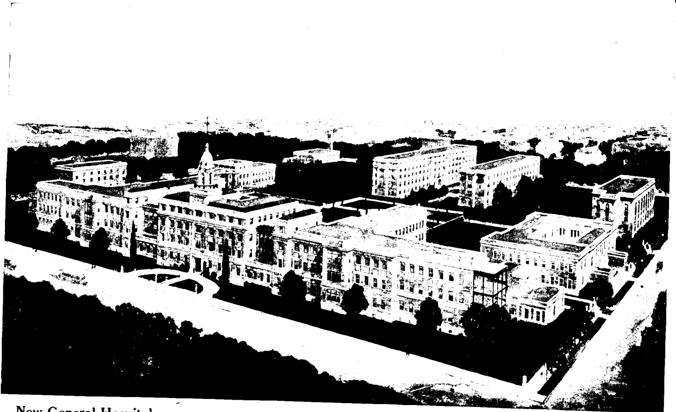
New General Hospital Toronto
