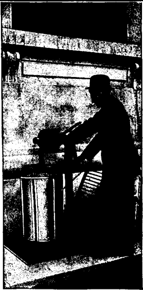
Hoist in Operation.
