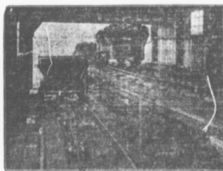
View of entrance to tippel showing loaded cars approaching the dump and empties on the return haul.
