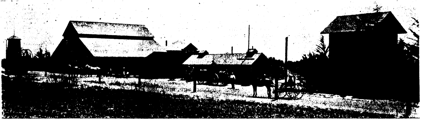
BUILDINGS ON G. B. REEVE'S RANCH, LA MIRADA, CALIFORNIA.
