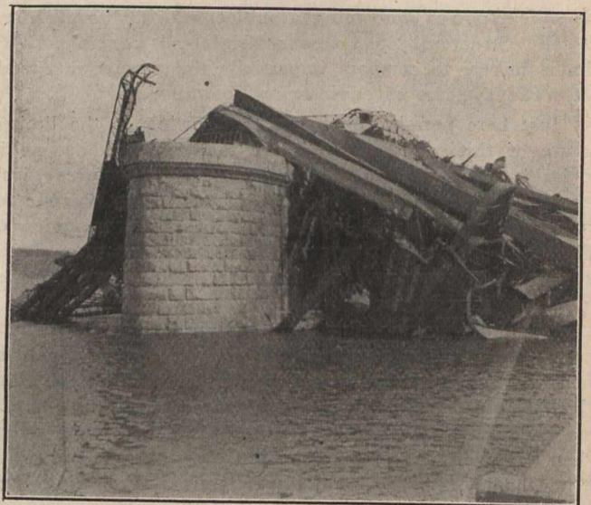
Fig. 2.—View of Main Pier after drop of nearly 400 feet.
