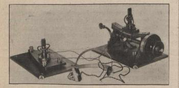
Telephonic Receiving-Mechanism of the Torsion Meter.
