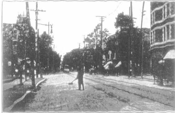
Concrete Road, Notre Dame Street E., Maisonneuve
