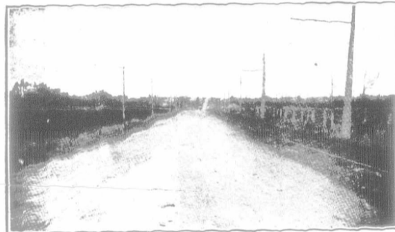
The Kingston Road in York County. Resurfaced with broken stones
