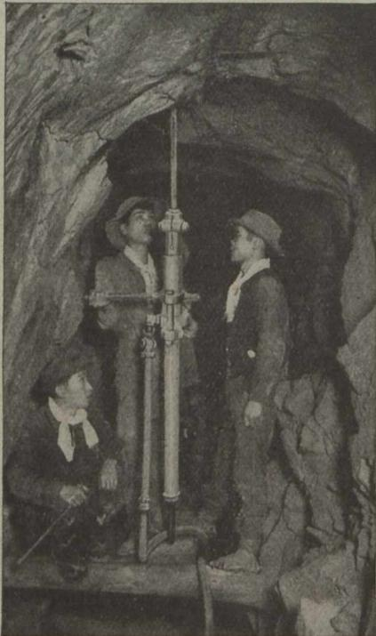
exactly suited to your needs. If your ground is soft or broken, choose "DF21" Light-hitting Stopers. If your ground is hard and tight, choose "DG21" Heavy-hitting Stopers. Then there's the "DA21" for average conditions, and the "DC21," with air jet, for flat holes. An atomizer, for laying dust, may be attached to any of these drills.
