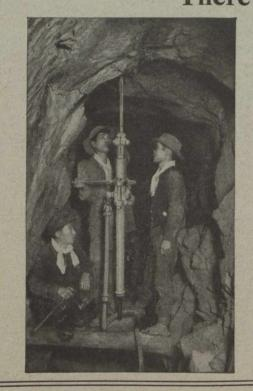
exactly suited to your needs. If your ground is soft or broken, choose "**DF21**" Light-hitting Stopers. If your ground is hard and tight, choose "**DG21**" Heavy-hitting Stopers. Then there's the "DA21" for average conditions, and the "DC21," with air jet, for flat holes. An atomizer, for laying dust, may be attached to any of these drills.
