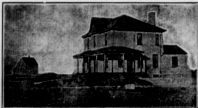
Superintendent's Residence, Nursery Station at Indian Head, 1905
