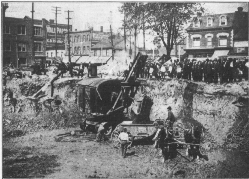
EXCAVATING FOR THE FOUNDATION OF THE NEW WESLEY BUILDINGS, JOHN STREETS, TORONTO.
