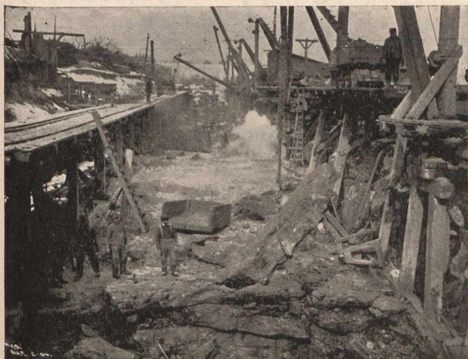
Toronto and Niagara Power Co.—Site of wheel pit in March, 1904.
