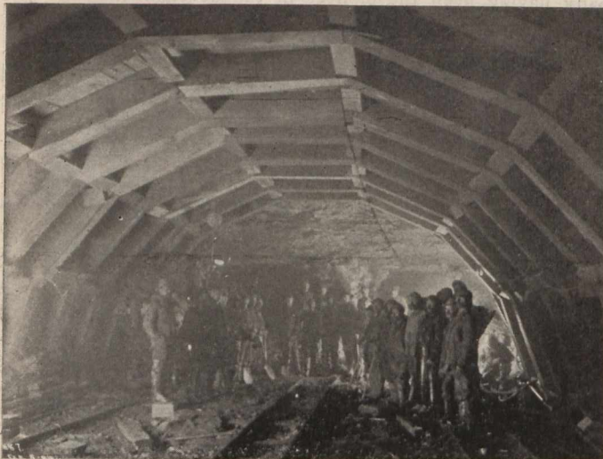
Toronto and Niagara Power Co.—View in tunnel.
