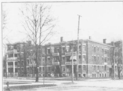
Apartment Houses, Queen's Ave.
