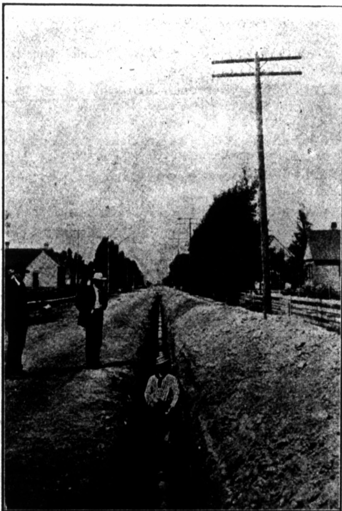
Showing our 14 inch Machine Banded Pressure Pipe being laid.
