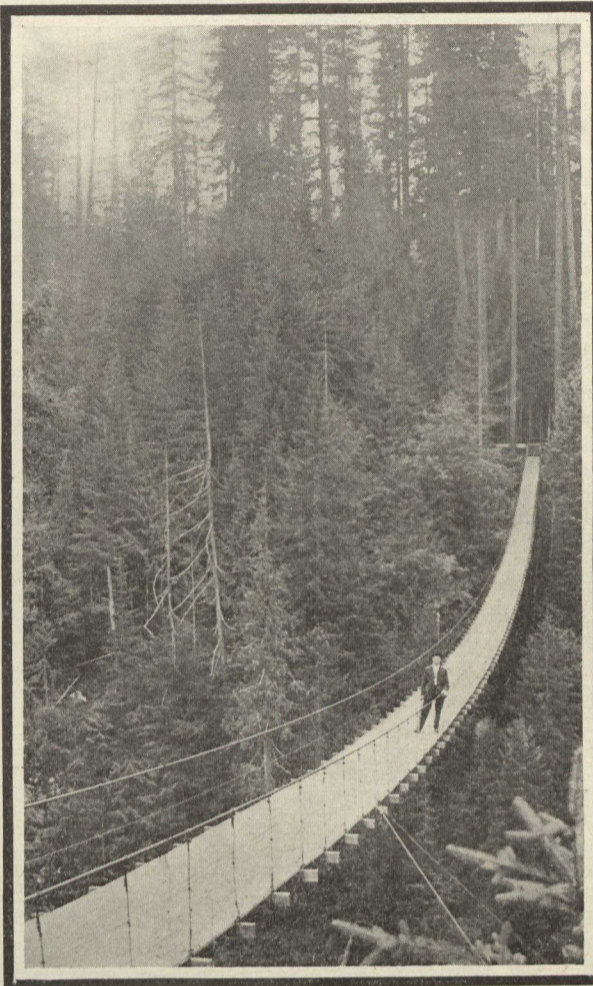
A Suspension Bridge swung amid the tree tops, spans the Capilano Canyon.
