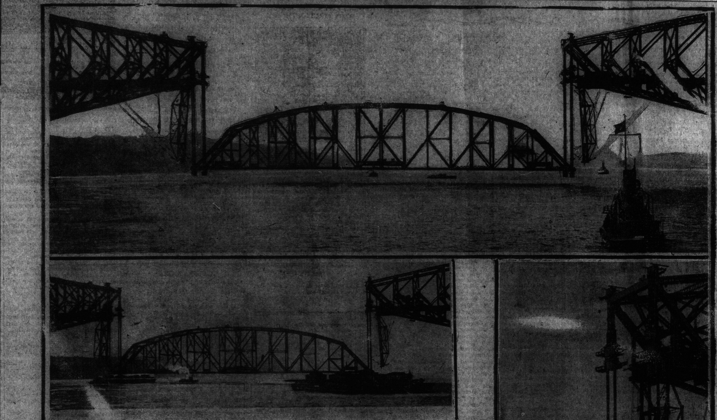
The picture immediately above shows the great span, floating on the scows, just after it was fixed into position, the mooring trusses at the side pulled back and the hoisting chains attached. The hydraulic jacks are seen on the lower level of the cantilever arms. The picture on the right shows the hydraulic jacks having lifted the span several feet towards its objective, while the central picture was taken after the span had disappeared in the waters of the St. Lawrence. The boat to the left of the chains is the government tug taking soundings in the channel, and finding that navigation will not be impeded by the mass of twisted metal lying 200 feet below the surface.
