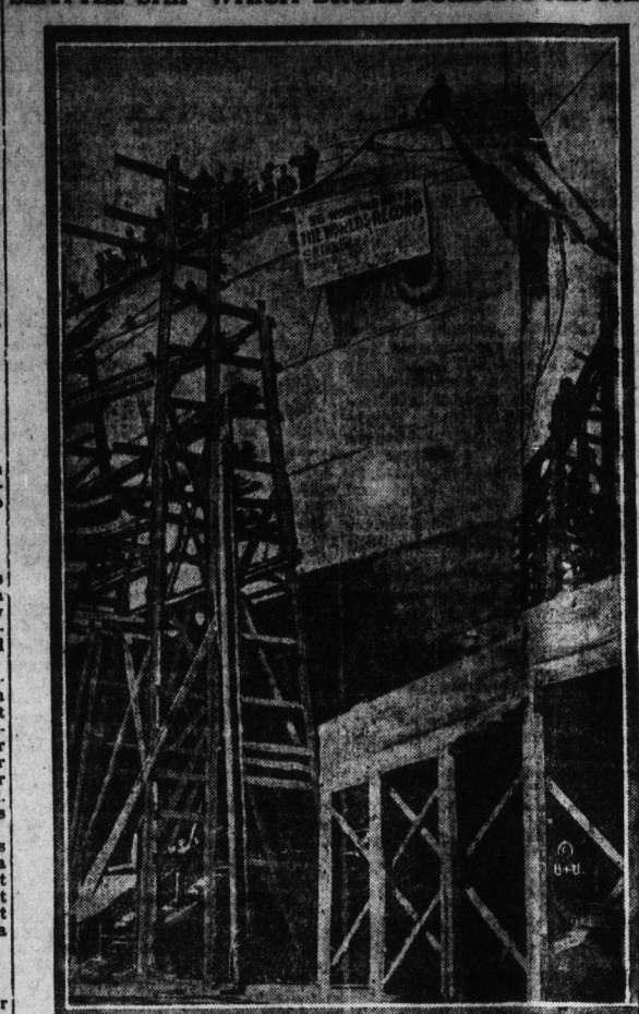
Fifty-five days after they laid the keel of the West Lianga, Skinner & Eddie, shipbuilders of Seattle, launched the vessel. In seventy-five days from the date of laying the keel the vessel will load cargo. Thus they made a record in the construction of a steel ship. If other shipbuilders work so rapidly it will not be long before Uncle Sam has sufficient ships to send an enormous army to the trenches.
