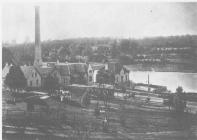
POWER HOUSE, WATERWORKS AND SPRINGBANK PARK.
