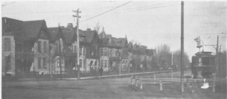
CENTRAL AVENUE, NORTH OF VICTORIA PARK, LOOKING EAST FROM RICHMOND STREET.
