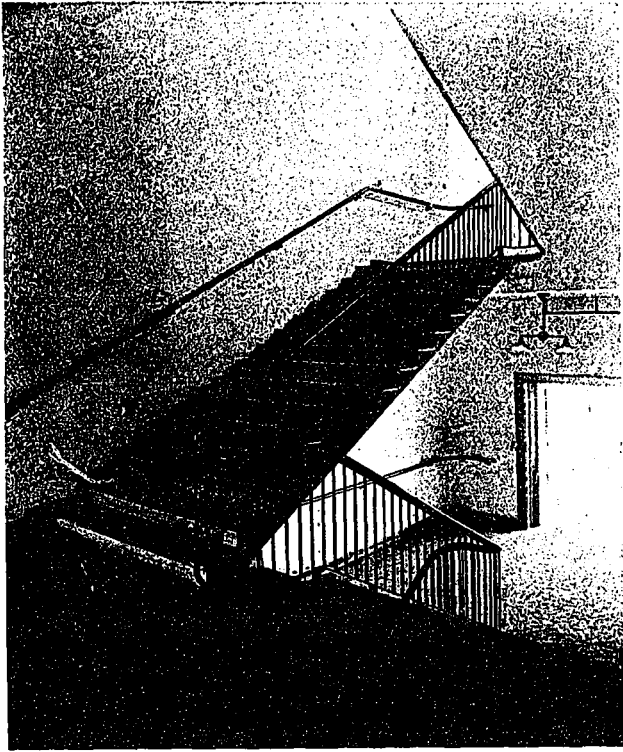
STAIRWAY, TODMORDEN SCHOOL.
