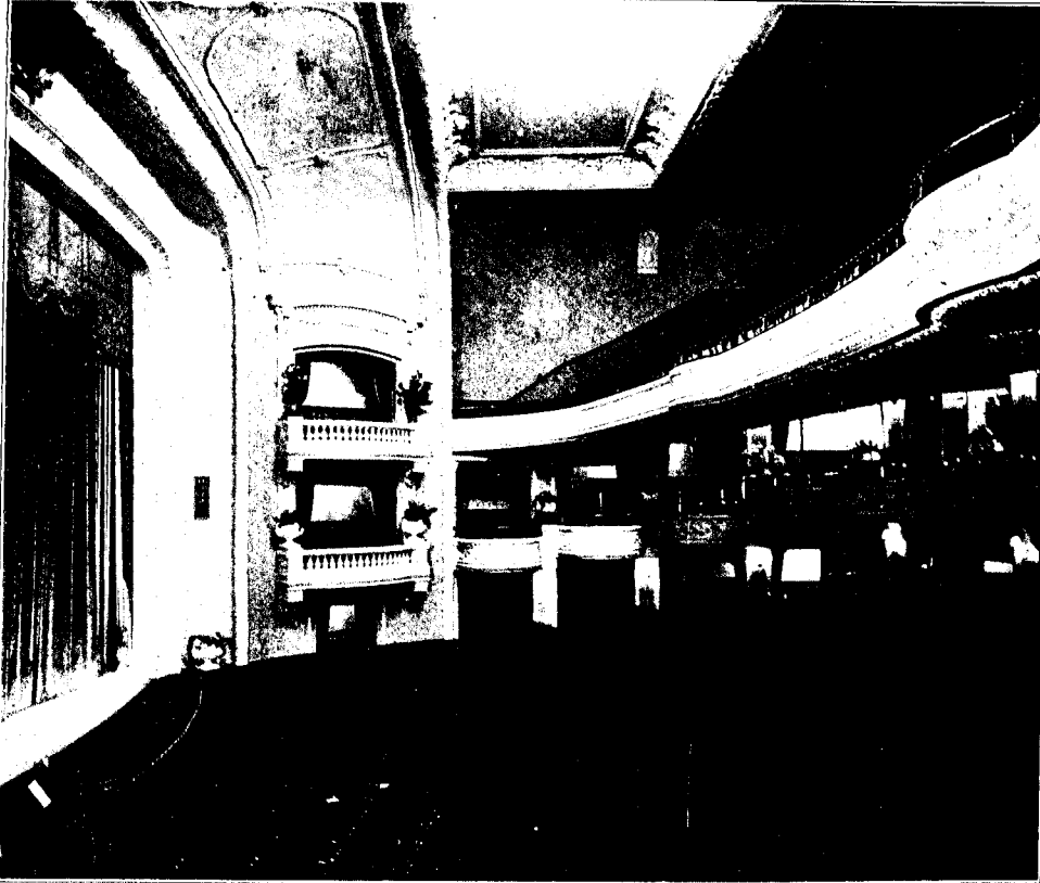
The Murray Theatre, Fort William, Ont. All the Lathing, Plastering and Ornamental Work was included in our Contract.
