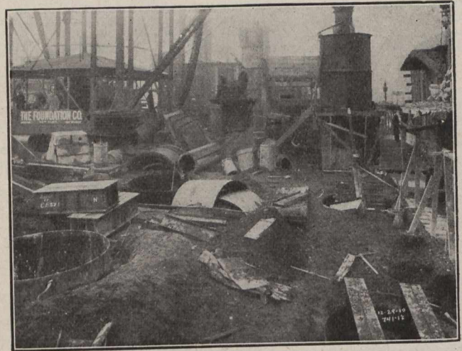
Fig. 4. Showing work on December 29, 1910, with grillage on Caisson in foreground.
