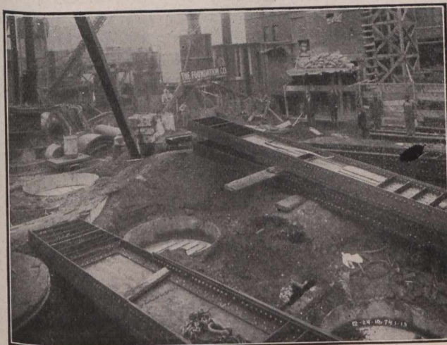
Fig. 5. On December 21, 1911, showing grillage concrete in place.
