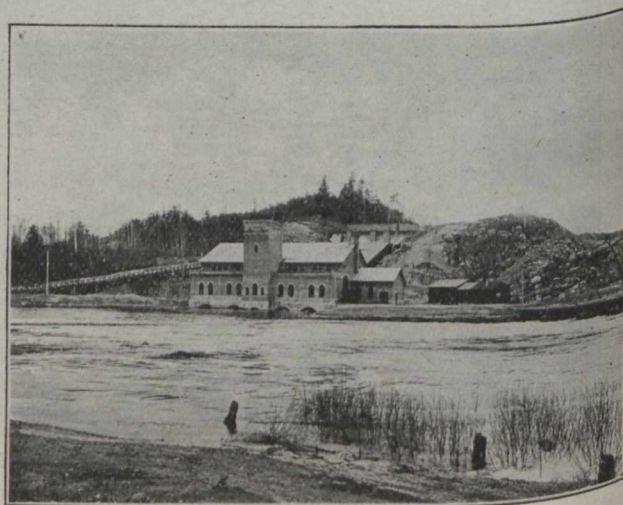
Power House at Crean Hill.
