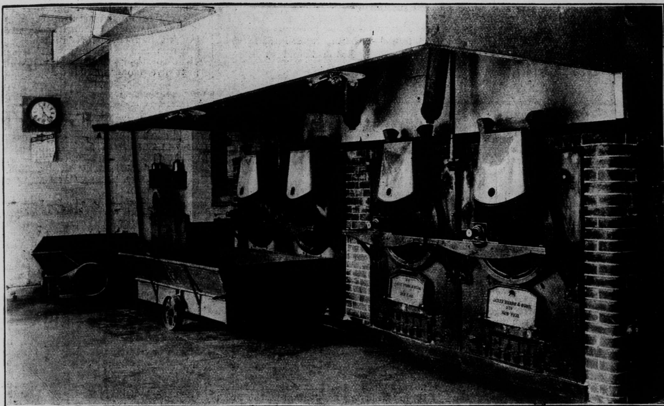
Battery of Roasters (incomplete) in Chase & Sanborn's New Factory. Two more Roasters to be installed.
