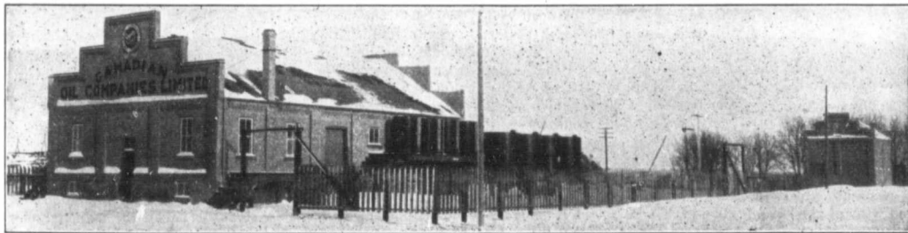
THE NEW PLANT OF THE CANADIAN OIL COMPANIES LIMITED, AT PORTAGE LA PRAIRIE
