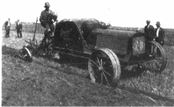
Emerson Brantingham 12-20 Model "L" Tractor, pulling an Emerson 3-furrow No. 2 Self-Lift Plow, with quick detachable Shares
