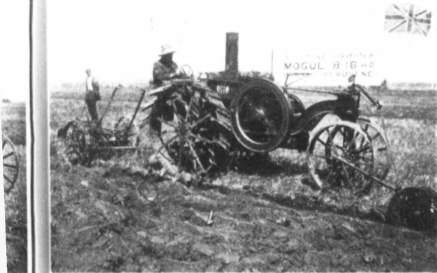
I. H. C. 8-16 Kerosene Tractor pulling a 3-furrow Oliver Plow
