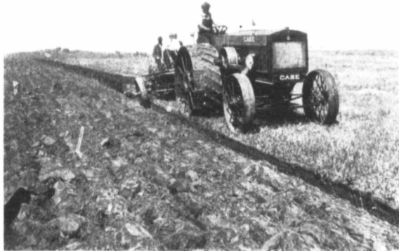
The Case 12-25 Tractor Pulling a 4-furrow Case Sattley Plow
