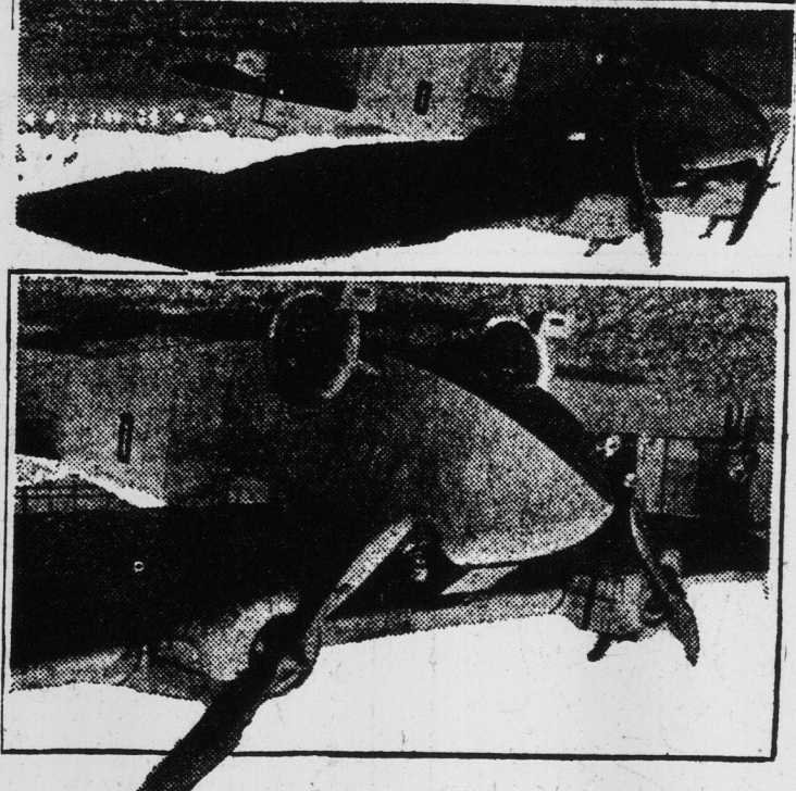
The latest in aeronautical design is incorporated in this new "flying Pullman" which has just gone into service between Berlin and other European capitals. This plane, a Junkers, has sleeping quarters for three as well as luxurious daytime accommodations for a number of passengers. Note the ingenious installation of the motors in the wing stream line, shown in the two views of the new plane.
