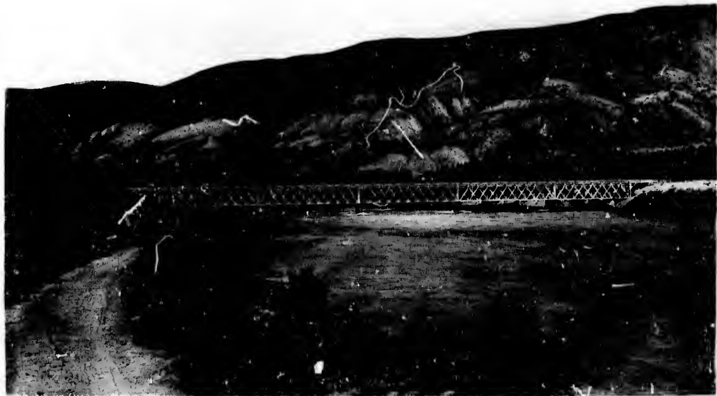
THOMPSON RIVER BRIDGE, ASHCROFT, B.C.
