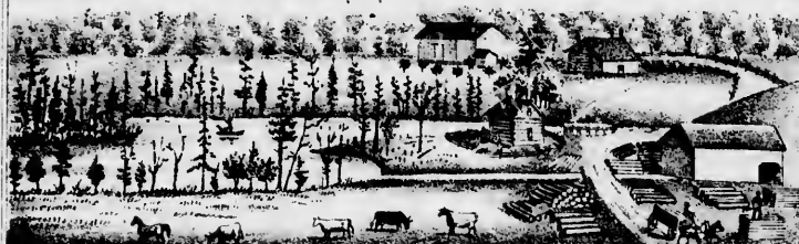
RES. A SAW MILL OF D. D. ROSS, CON 1, LOTS 25, 26, 27 & 28, KINLOSS T h BRUCE CO. ONT
