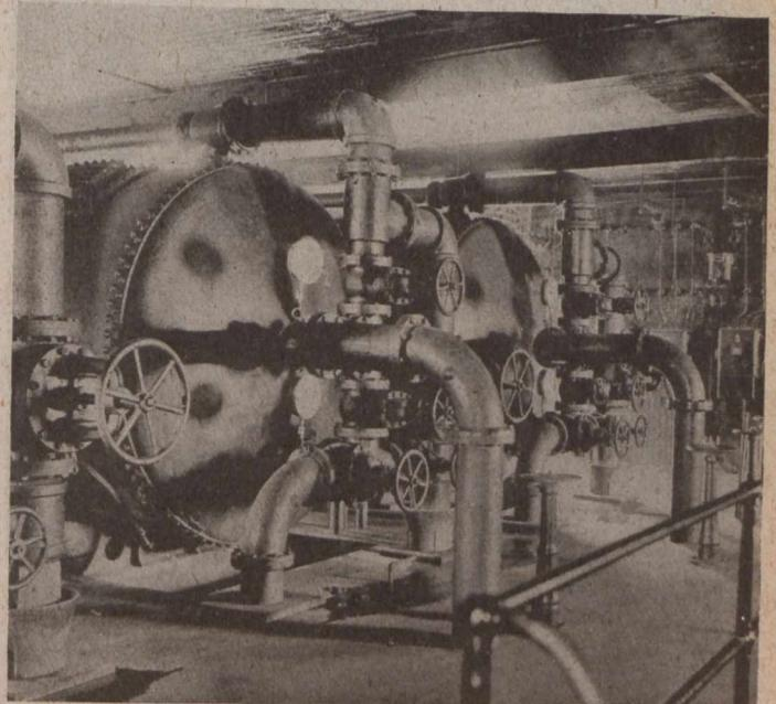
FIG. 2—MECHANICAL FILTER TANKS
