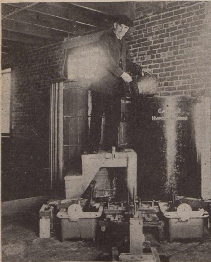
FIG. 3—AUTOMATIC DEVICE DESIGNED BY THE "HYDRO" MUNICIPAL ENGINEERING STAFF FOR FEEDING COAGULANT AND HYPOCHLORITE
