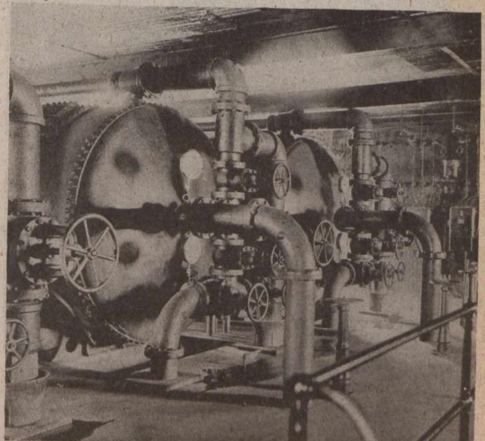
FIG. 2—MECHANICAL FILTER TANKS
