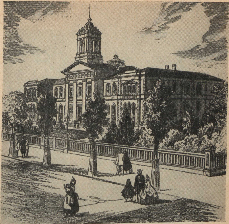
NORMAL SCHOOL BUILDINGS, TORONTO
