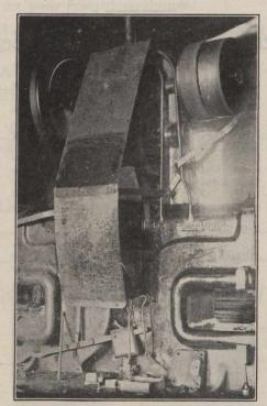
Fig. 2.—Gear Protection on Punch Press.
