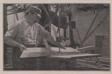
Sawing Pilot Slats to Shape on the Band Saw.
