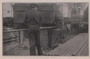
Fig. 7 .- Swedging First Tube Ends.
