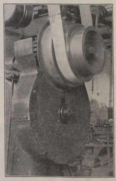
Fig. 1.—Gear Protection on a Slotter.
