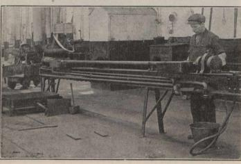
Fig. 9 .- Testing Safe-ended Tube.
