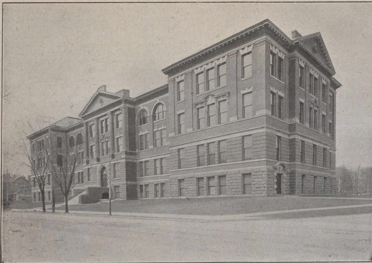
The Chemical and Mining Building
