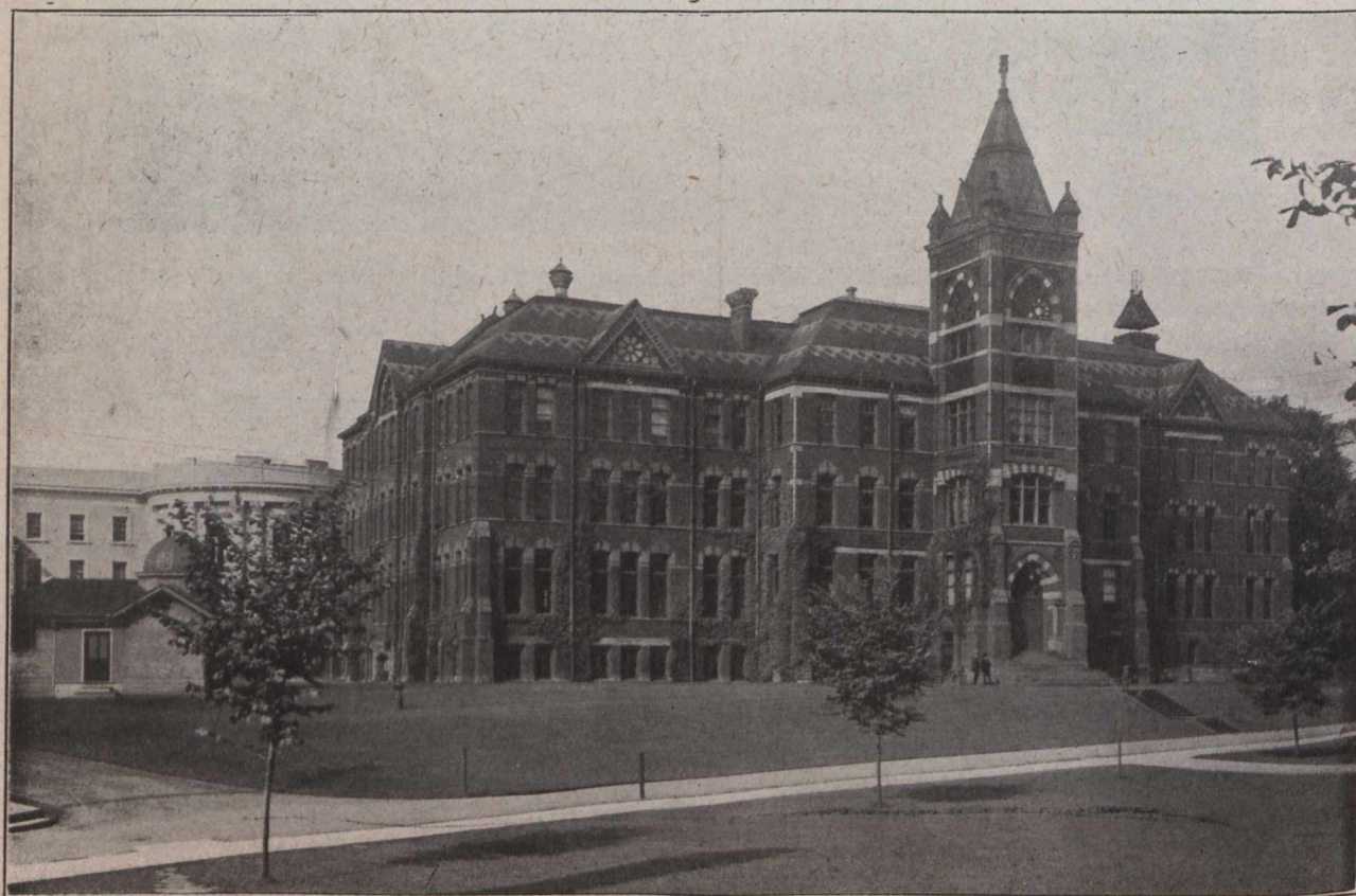
Main Engineering Building, The Old S.P.S.
