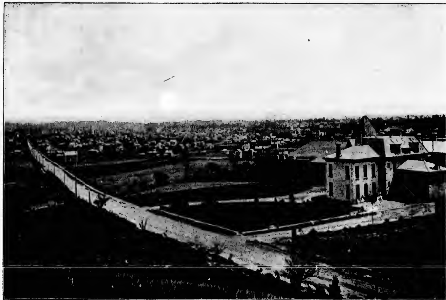
VIEW FROM THE STAND PIPE.
