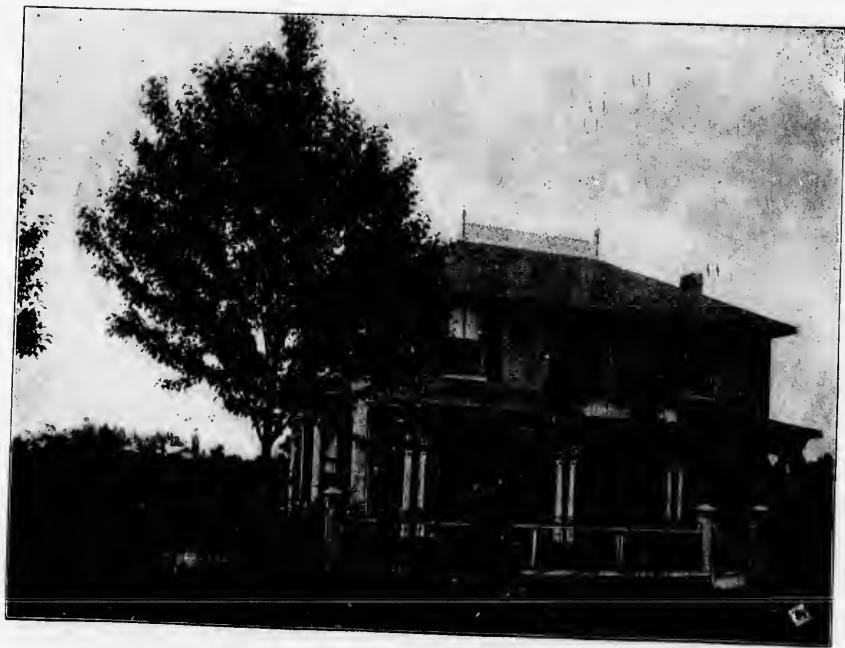
W. T. WALKER'S RESIDENCE, McKenzie Street.
