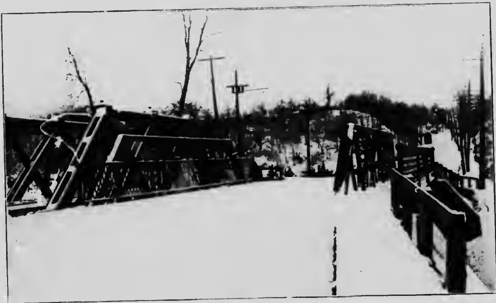
WESTON ROAD BRIDGE OVER BLACK CREEK, TOWNSHIP OF YORK.
