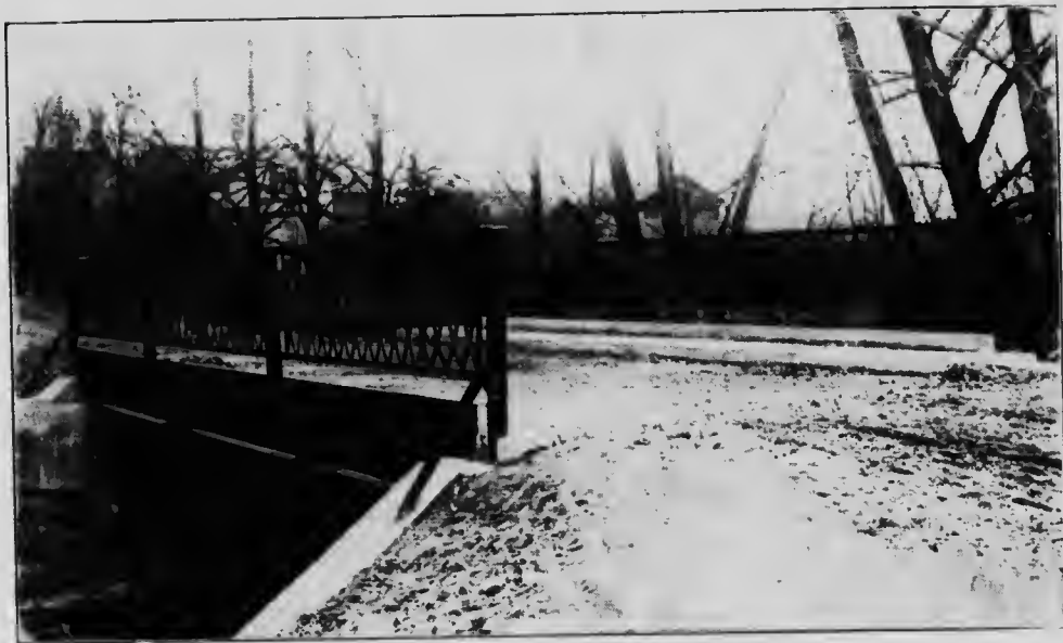
SRIGLEY STREET BRIDGE, NEWMARKET, ONT.
