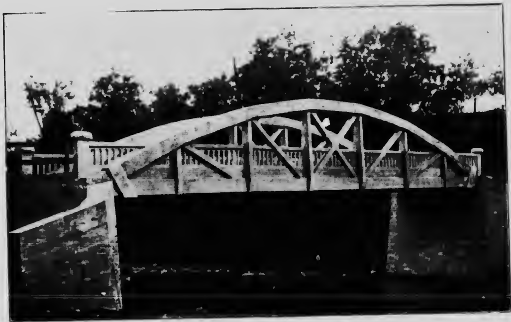
MIDDLE ROAD BRIDGE.
