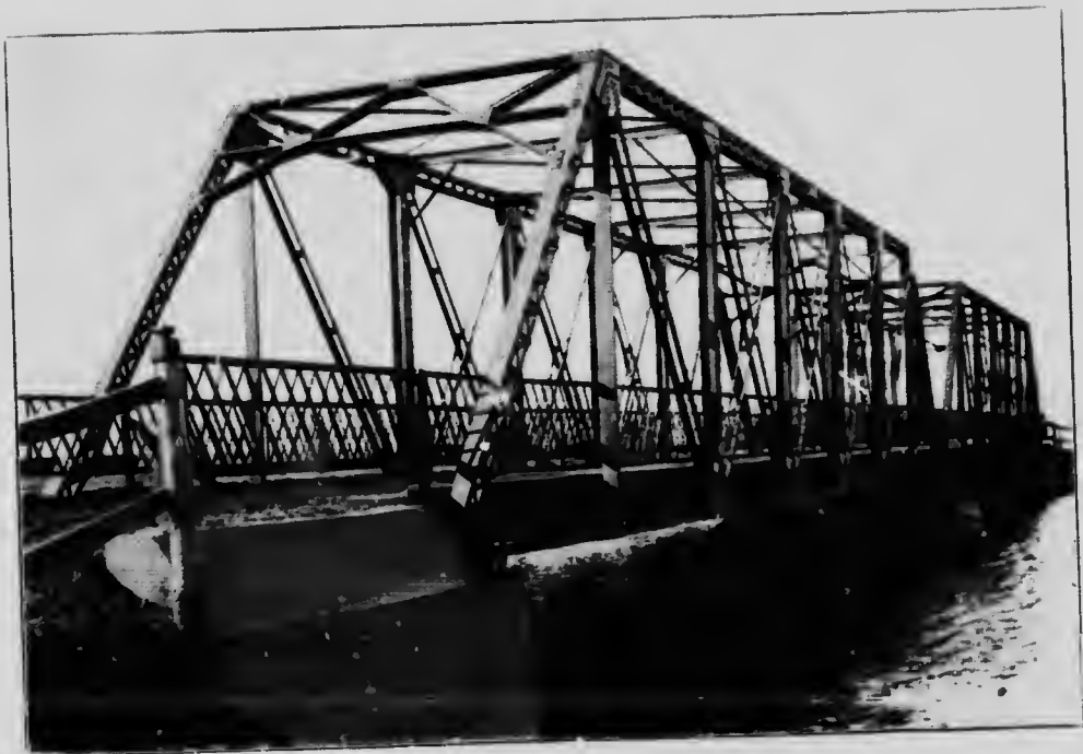
BRIDGE OVER HOLLAND RIVER, NEAR BRADFORD, ONT.
