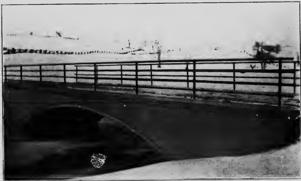
BRIDGE ON TOWNLINE BETWEEN KING AND VAUGHAN TOWNSHIPS, COUNTY OF YORK.
