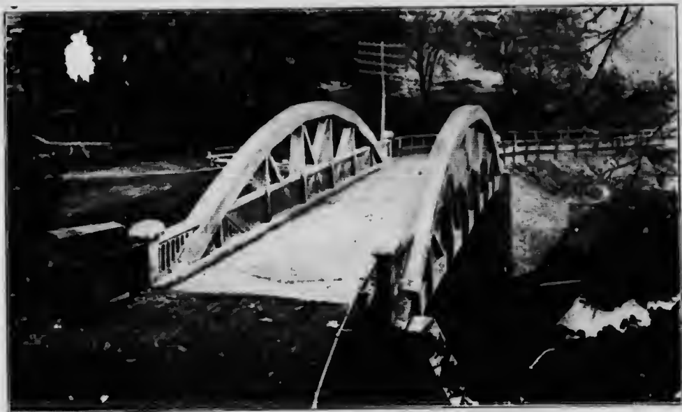
MIDDLE ROAD BRIDGE.
