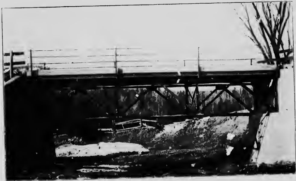
BRIDGE OVER HIGHLAND CREEK, TOWNSHIP OF SCARBORO'.
