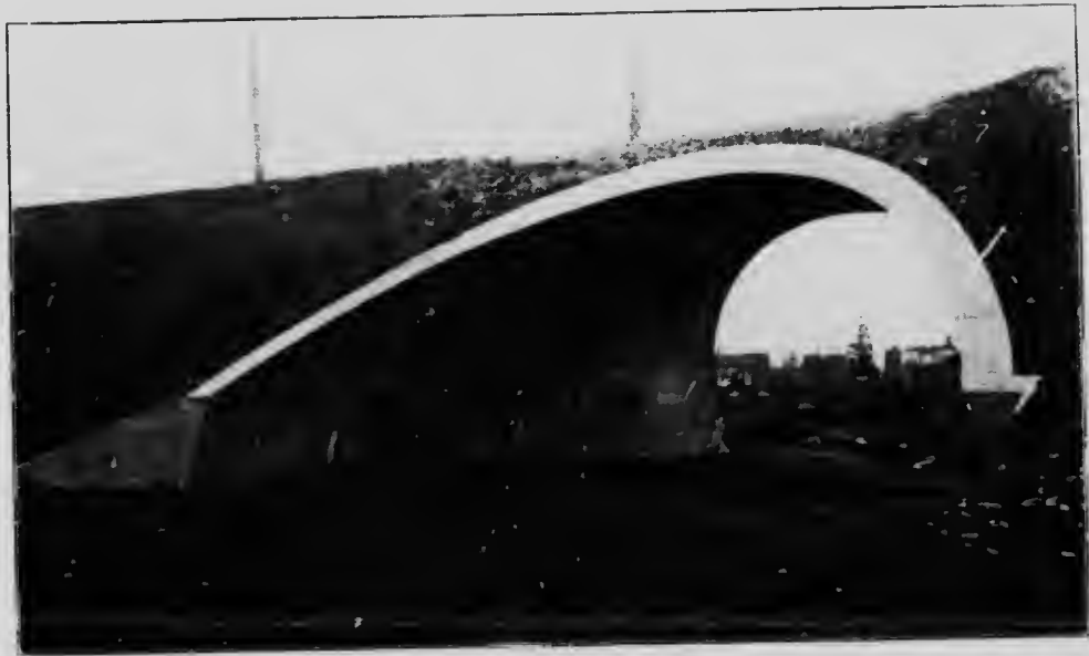
ARCH OVER HOLLAND RIVER, NEWMARKET, ONT.
