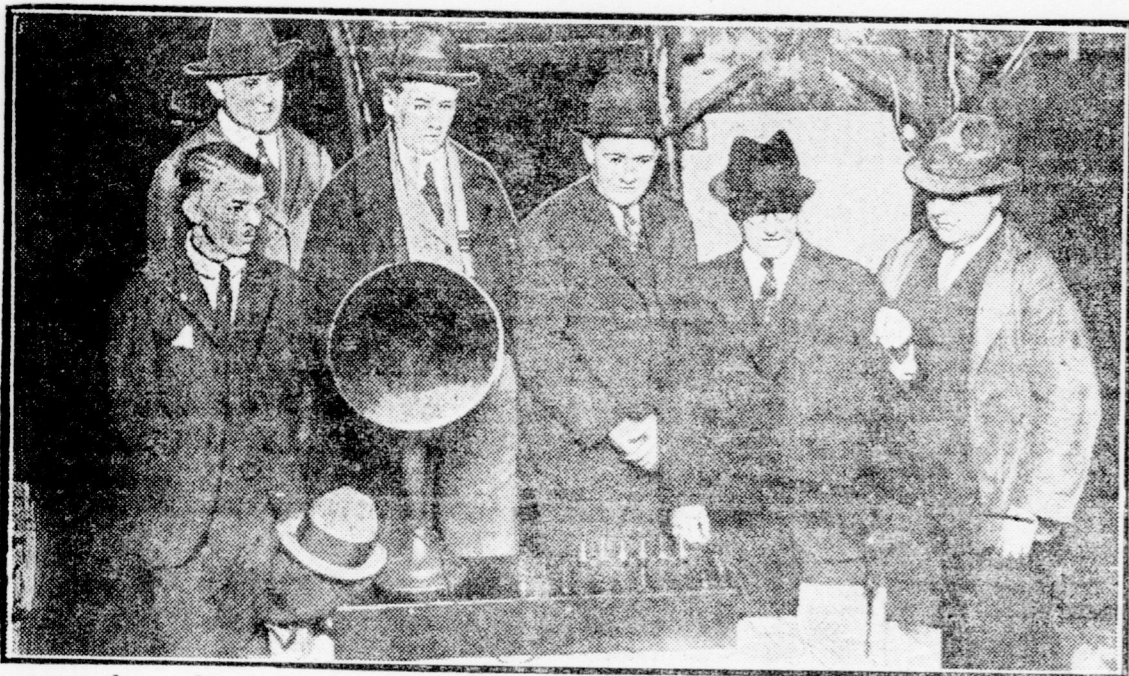
In a tunnel, one hundred feet under the surface of the Hudson River, engineers and newspaper men listened to a radio test from Pittsburg. The waves traveled through 500 miles of air, 70 feet of water and 30 feet of mud and steel casing
